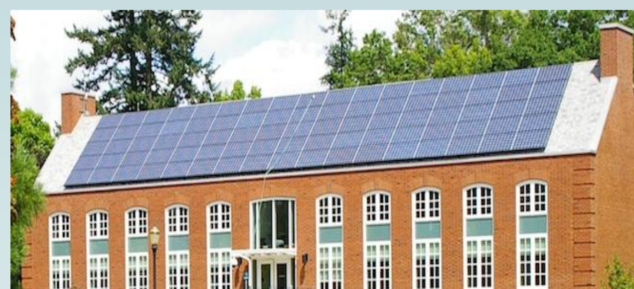
Figure 1: Solar Cells on TJ Day Hall of Linfield College, McMinnville Campus
