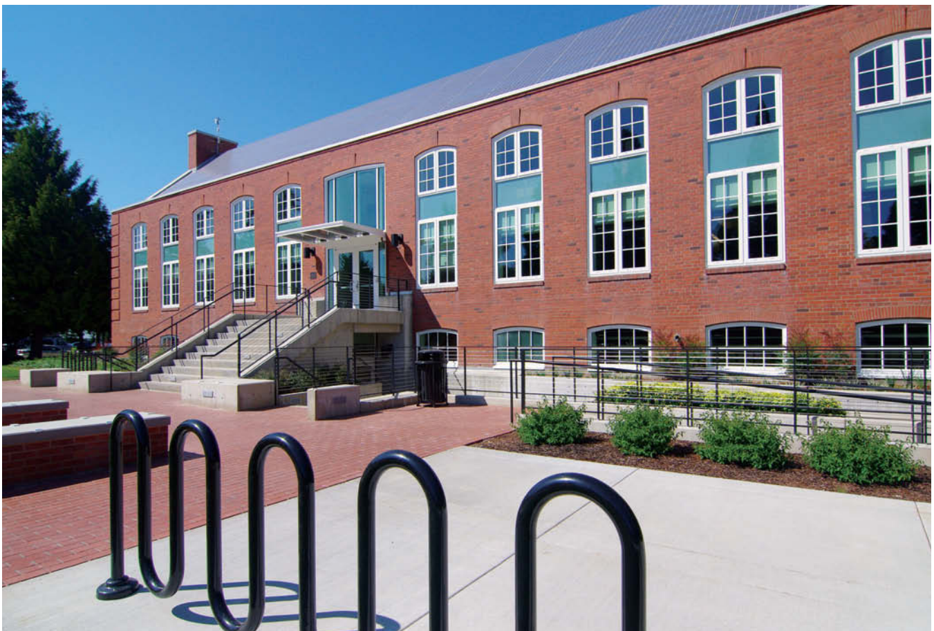
Top, construction phase in entryway and at the south entrance. Bottom, new south entrance off the Academic Quadrangle.
